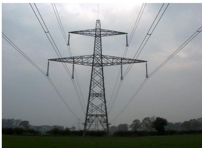
Image 5.14 Typical low height lattice pylon (suspension (left) and tension pylon (right)) 4 (source: Land Use Consultants, 2024)
