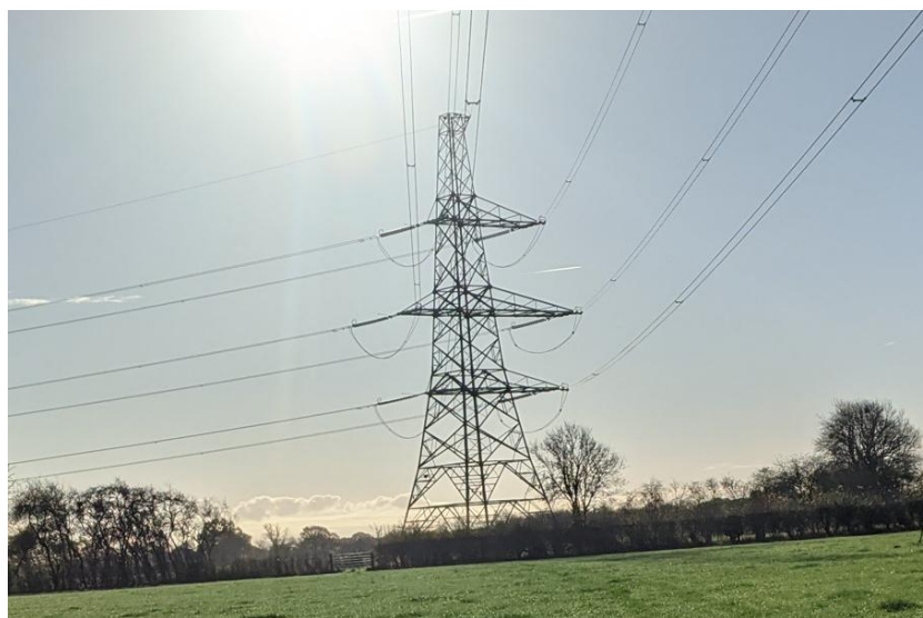
Image 5.12 Typical tension/angle lattice pylon 2
