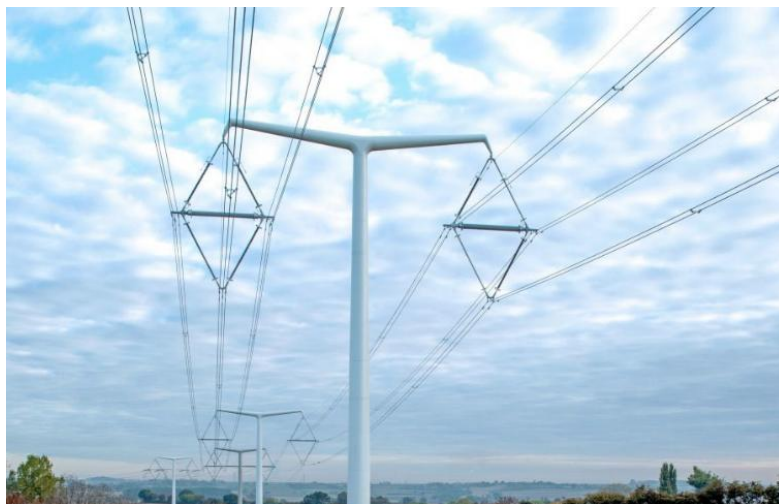
Image 5.9 Typical suspension T-pylon
