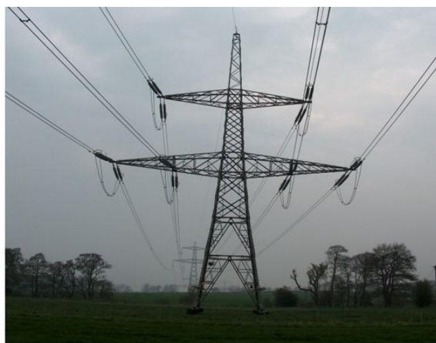
Image 5.14 Typical low height lattice pylon (suspension (left) and tension pylon (right)) 4 (source: Land Use Consultants, 2024)
